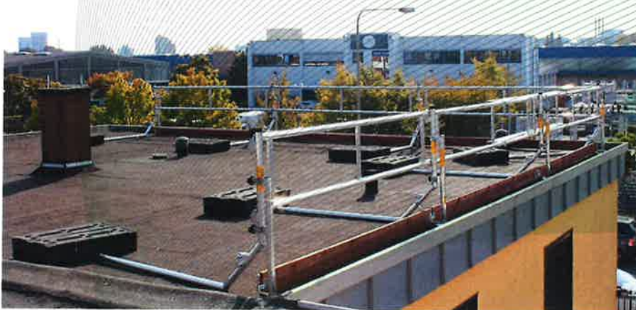
Fig. 1: Edge protection system, type: flat roof railing system
